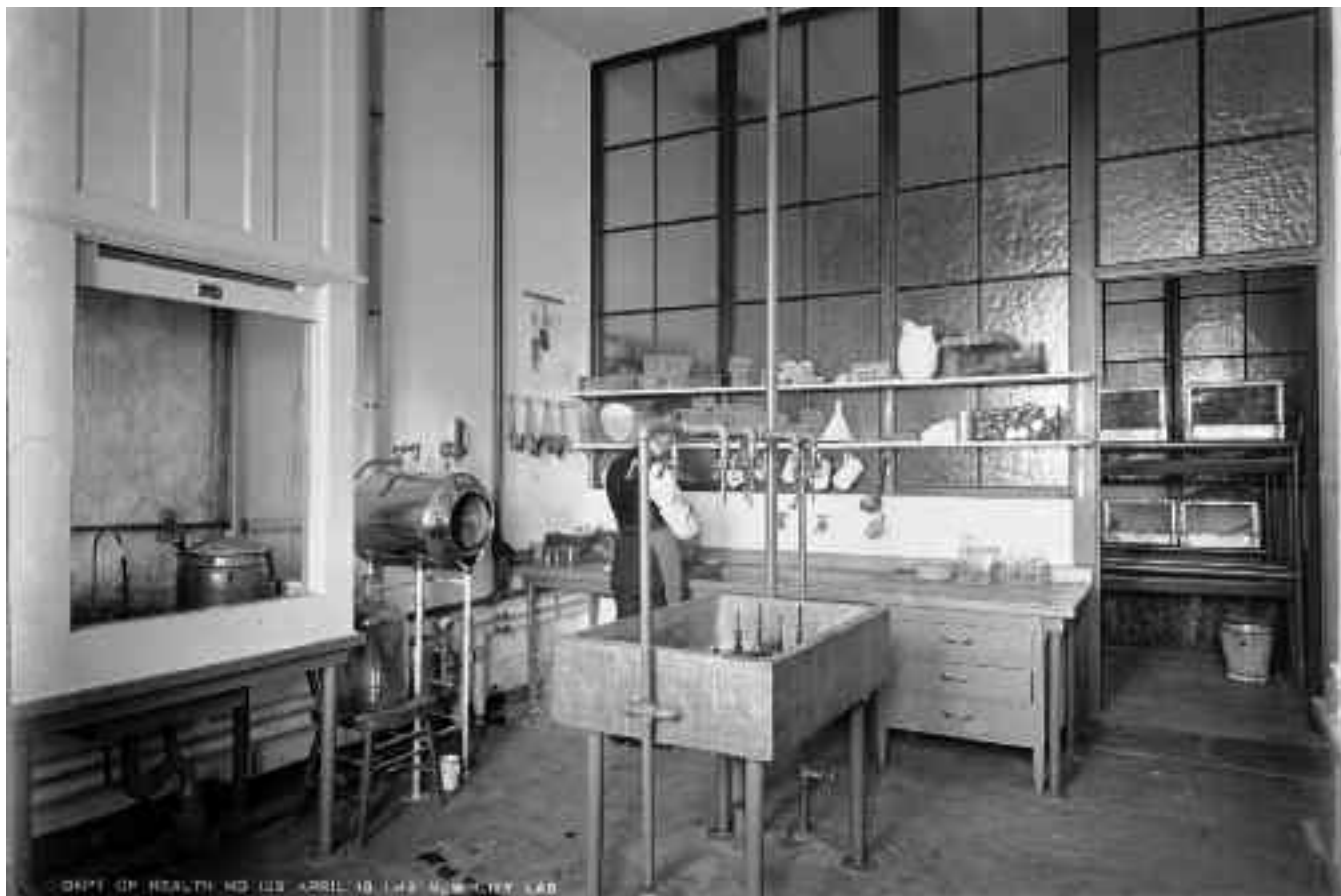
Figure 4. In contrast, Toronto's new City Laboratory, opened in 1912, shines with science. The camera focuses on the dedicated area for milk analysis with its own plumbing and lighting, the centrifuge, and the animal cages behind. Stainless steel equipment and fixtures have replaced wooden fittings, and the sole technician wears laboratory garb. (City of Toronto Archives)
